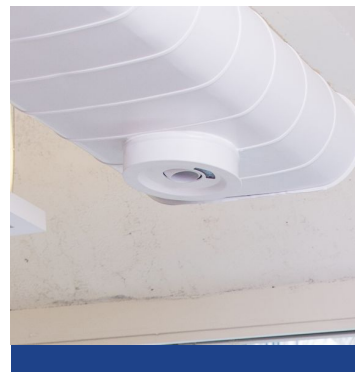
Exposed Metal Duct Page 15
