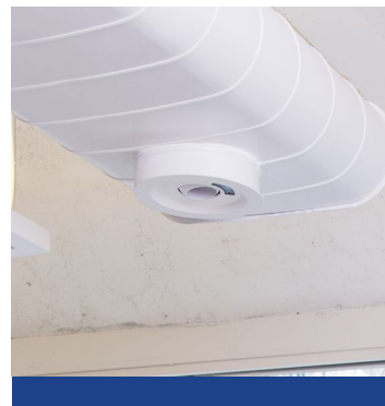
Exposed Metal Duct Page 15
